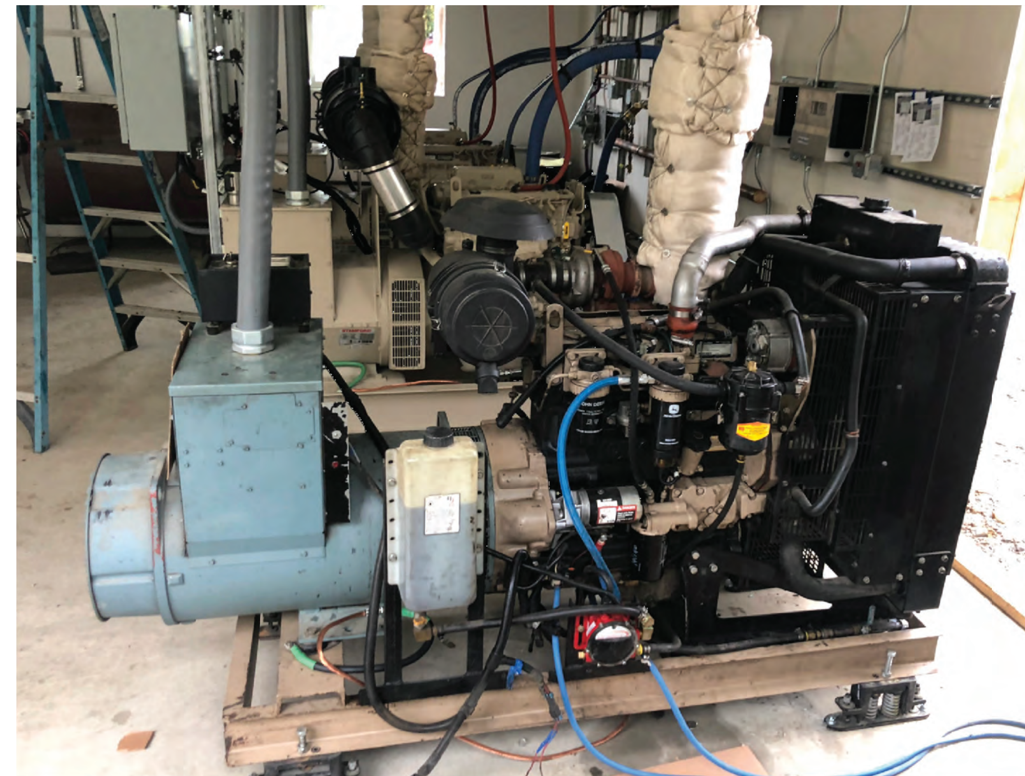
4 EXISTING GEN#3 REFERENCE PHOTO ER2 1"=1'-0"
