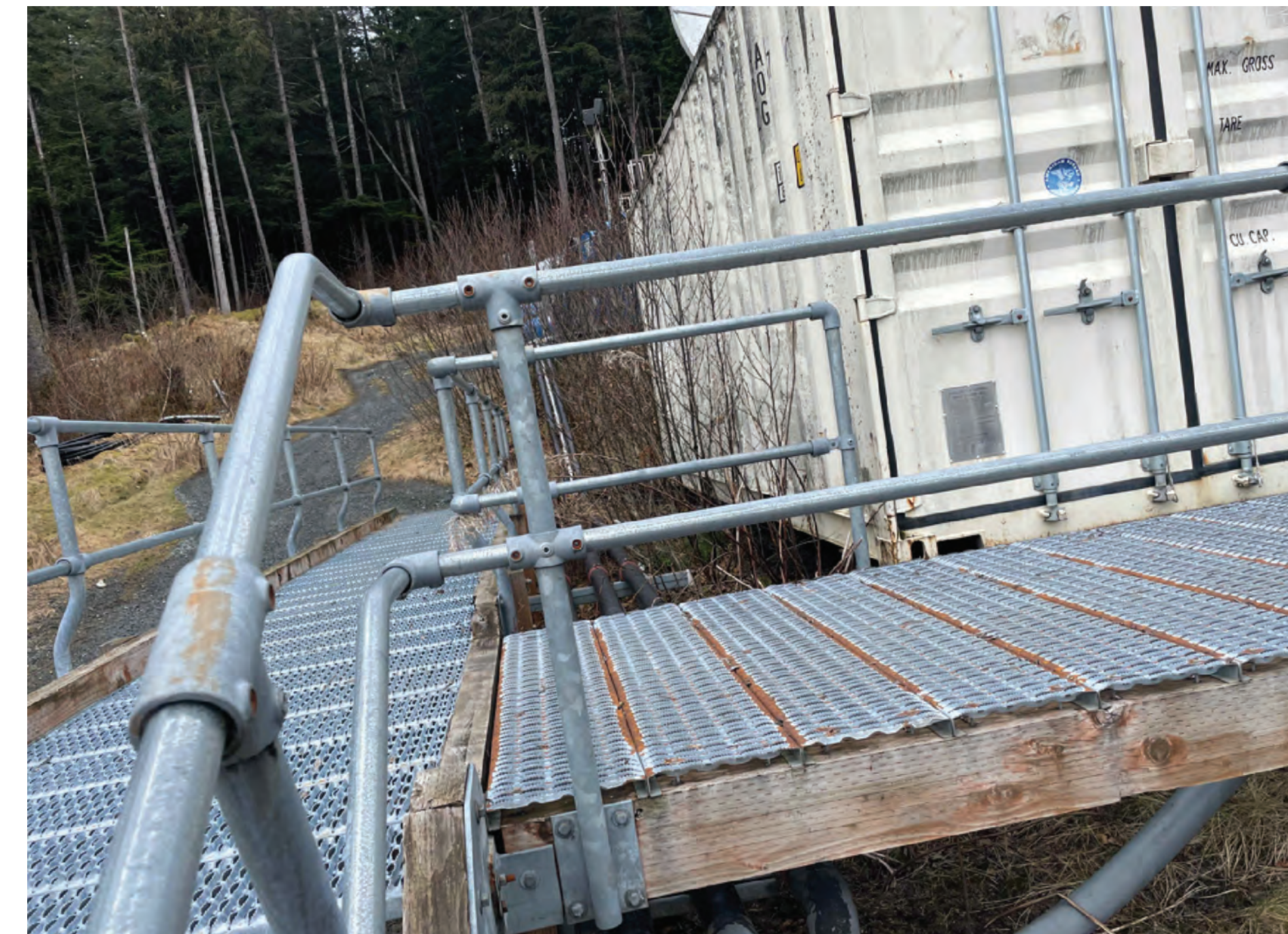
4 PHOTO 2 - CATWALK FOR GENERATOR ACCESS NO SCALE
