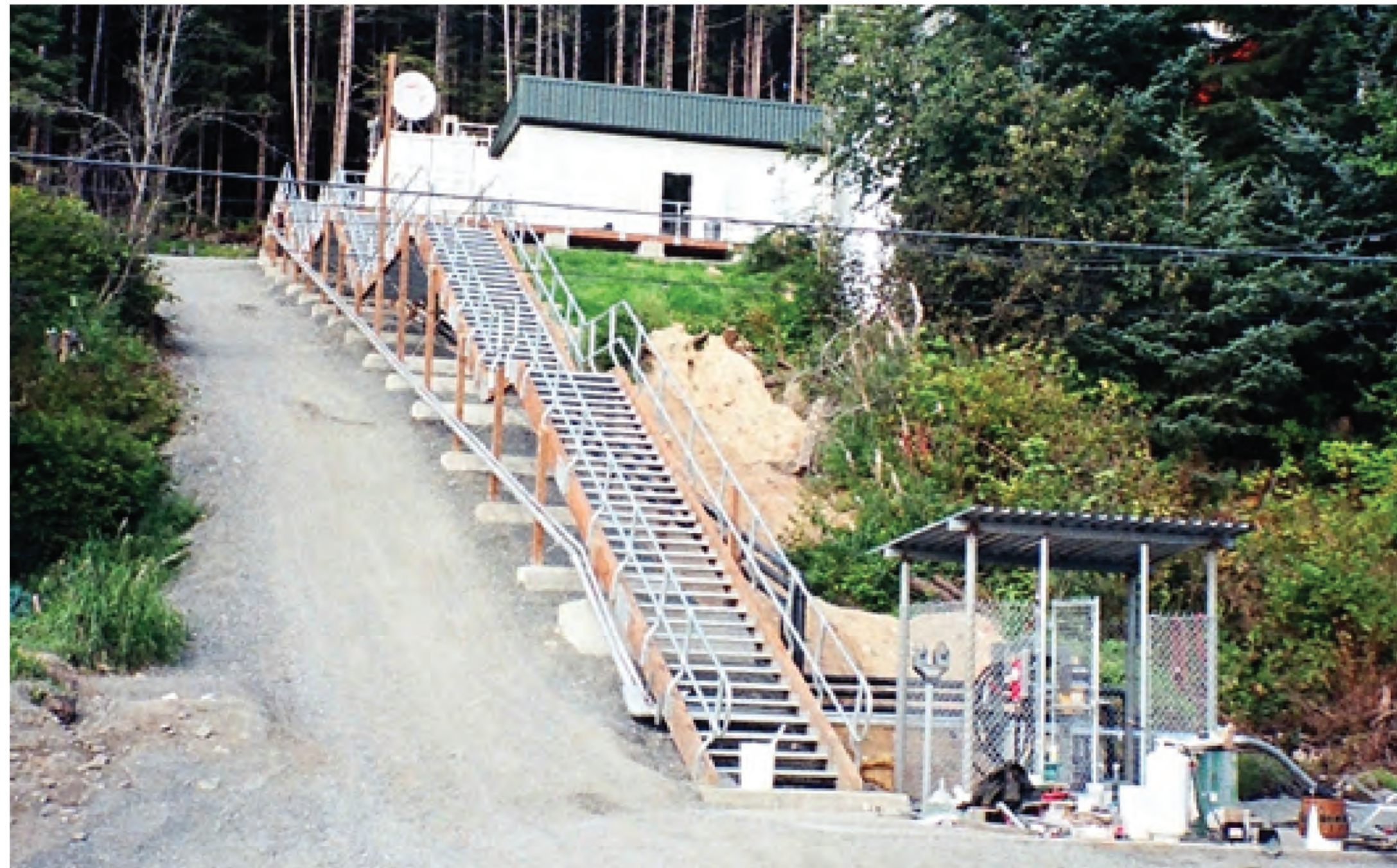
3 PHOTO 1 - ACCESS ROAD & STAIRS NO SCALE
