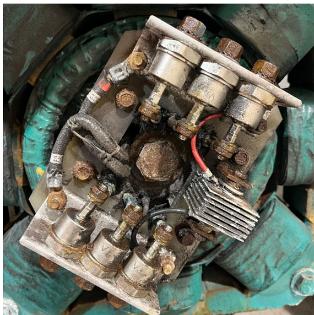
Rectifier assembly needing replacement.
