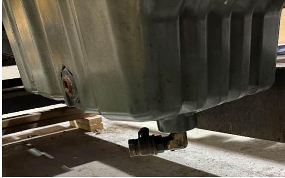
Overview from left rear. Note dented enclosure.
