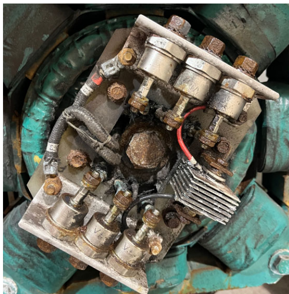
Rectifier assembly needing replacement.
