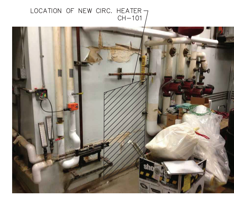
B CIRCULATION HEATER MOUNTING LOCATION SCALE: N.T.S.
