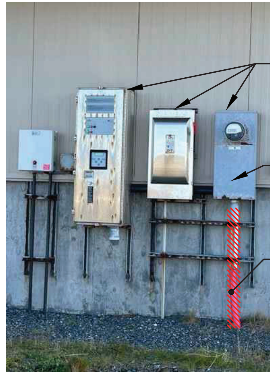
ICE HOUSE 480v 3Ø SERVICE DEMOLITION
