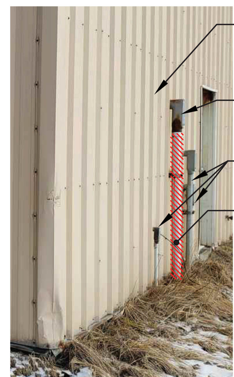
STORAGE COMPOUND 480v 3Ø SERVICE DEMOLITION
