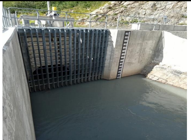
Photo 22 – Spillway Drain – Photo from AEA
