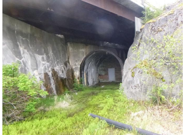
Photo 14 – Penstock Tunnel Outlet
