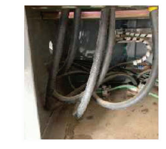
EXISTING FLOOR PENETRATION
