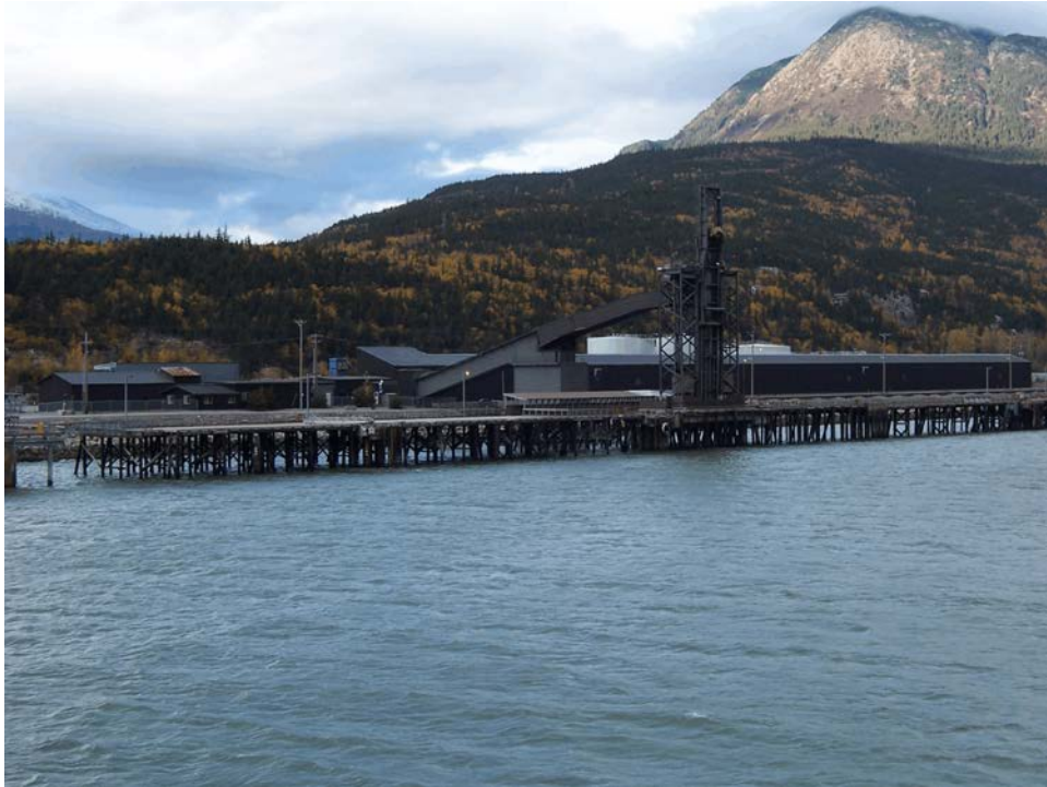
Overview of subject property from ferry terminal looking northwest.
