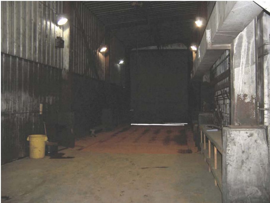
Interior of equipment wash building.
