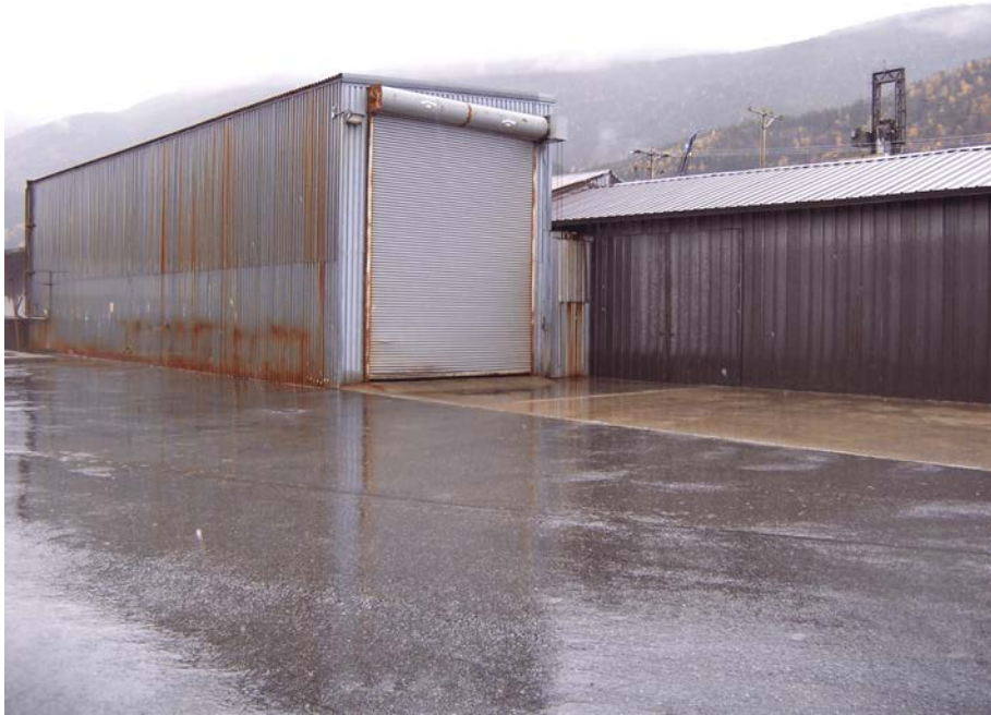
Equipment wash building photo left tied in to maintenance shop photo right.
