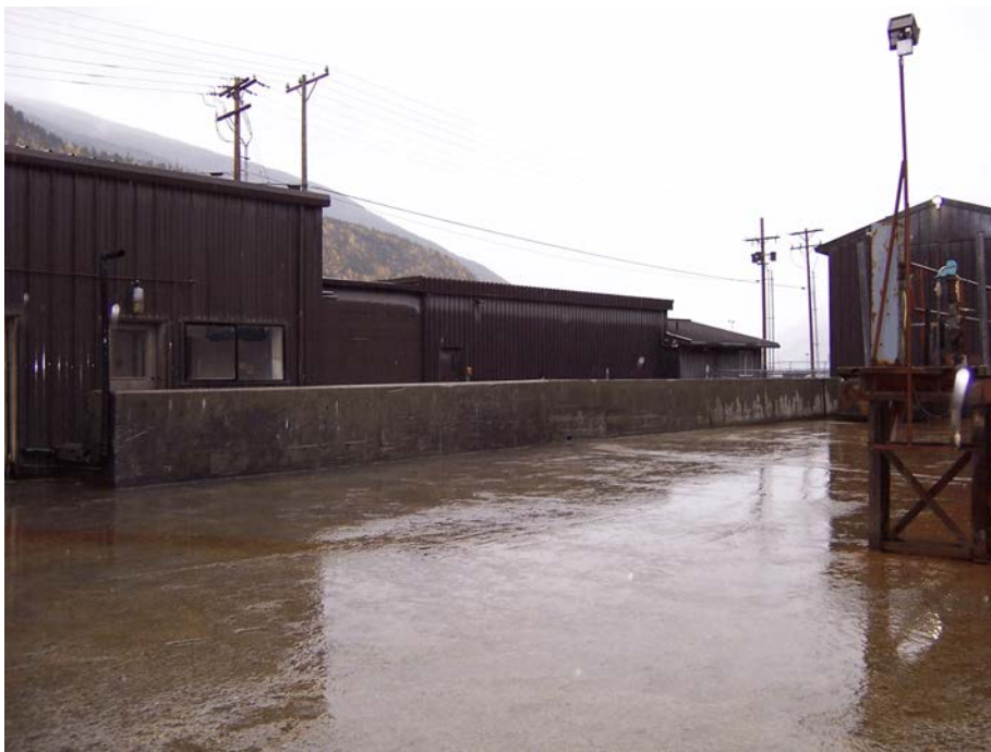
Looking southeast across the equipment parking and wash area; 101105_2324 laboratory building photo left and combination of electric transformer, crew changing, office building photo center, and maintenance shop photo right.
