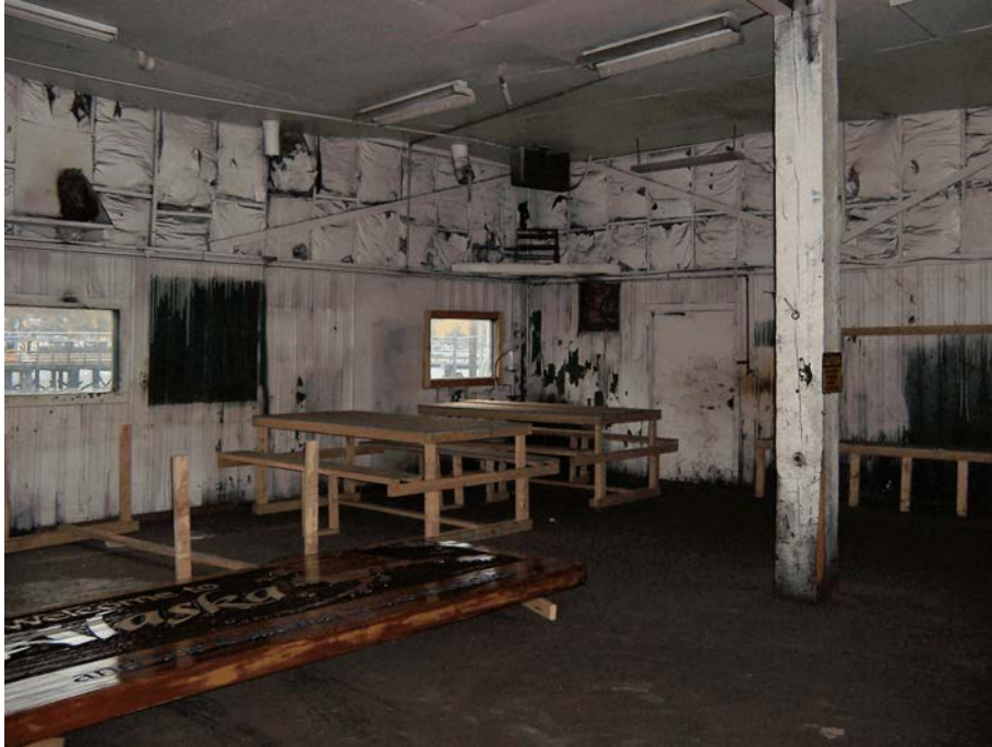
Interior of maintenance shop building.
