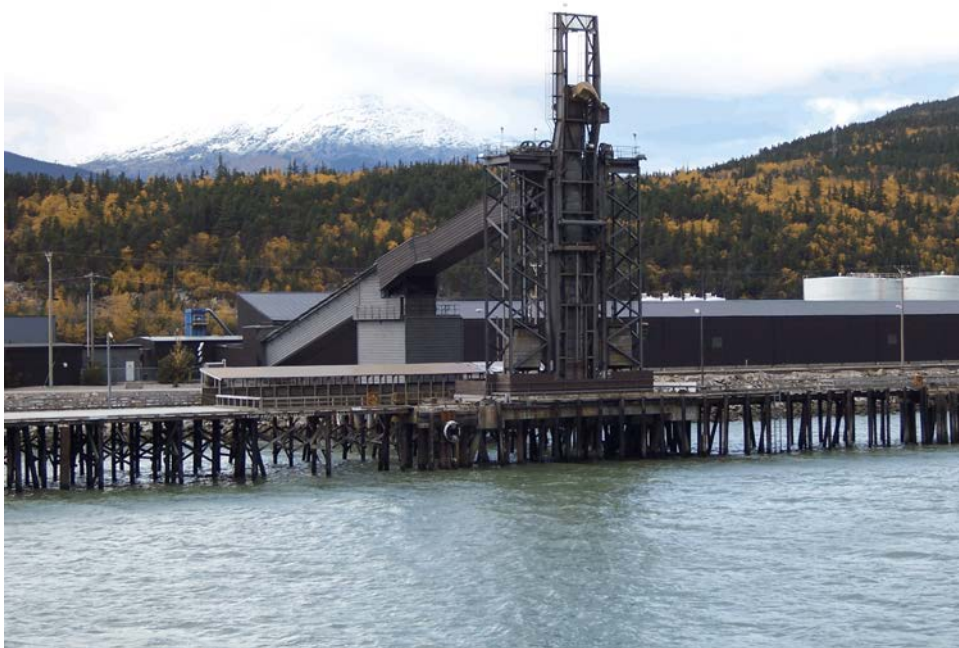
Shiploading conveyor system.
