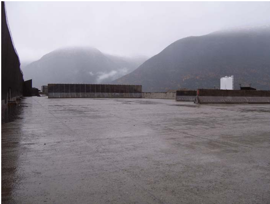
Looking in a south to southwest direction across the storage area.
