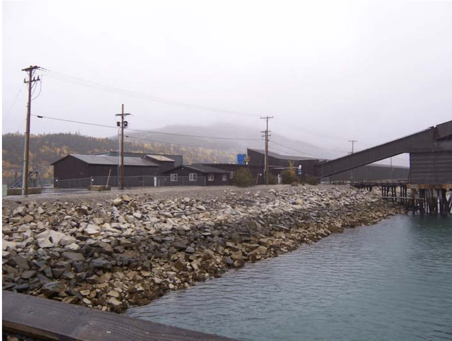
Southern end of subject property looking northwest at miscellaneous 101105_2331 buildings. Maintenance shop building photo left. Office building small one-story photo center with crew changing building attached and directly behind that building. Transfer conveyor system photo right ties into the laboratory building.
