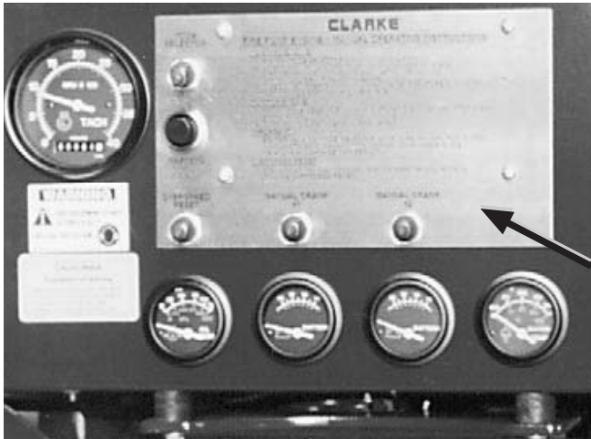
Fig. 2 - Emergency Operating Instructions
