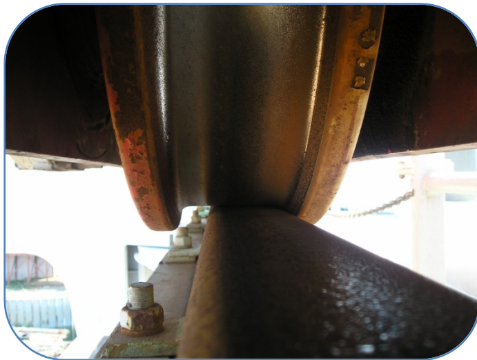
Figure 1 – Looking Down the Landside Rail
