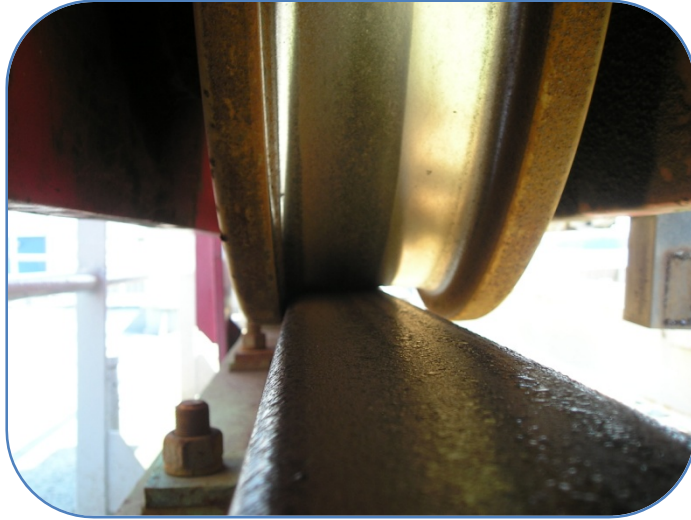
Figure 2 – Looking Down the Waterside Rail
