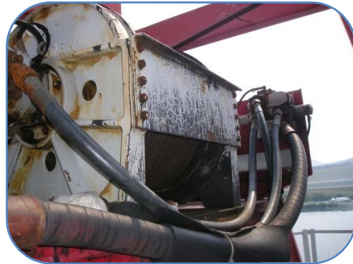
Main Hoist (Load) Winch
