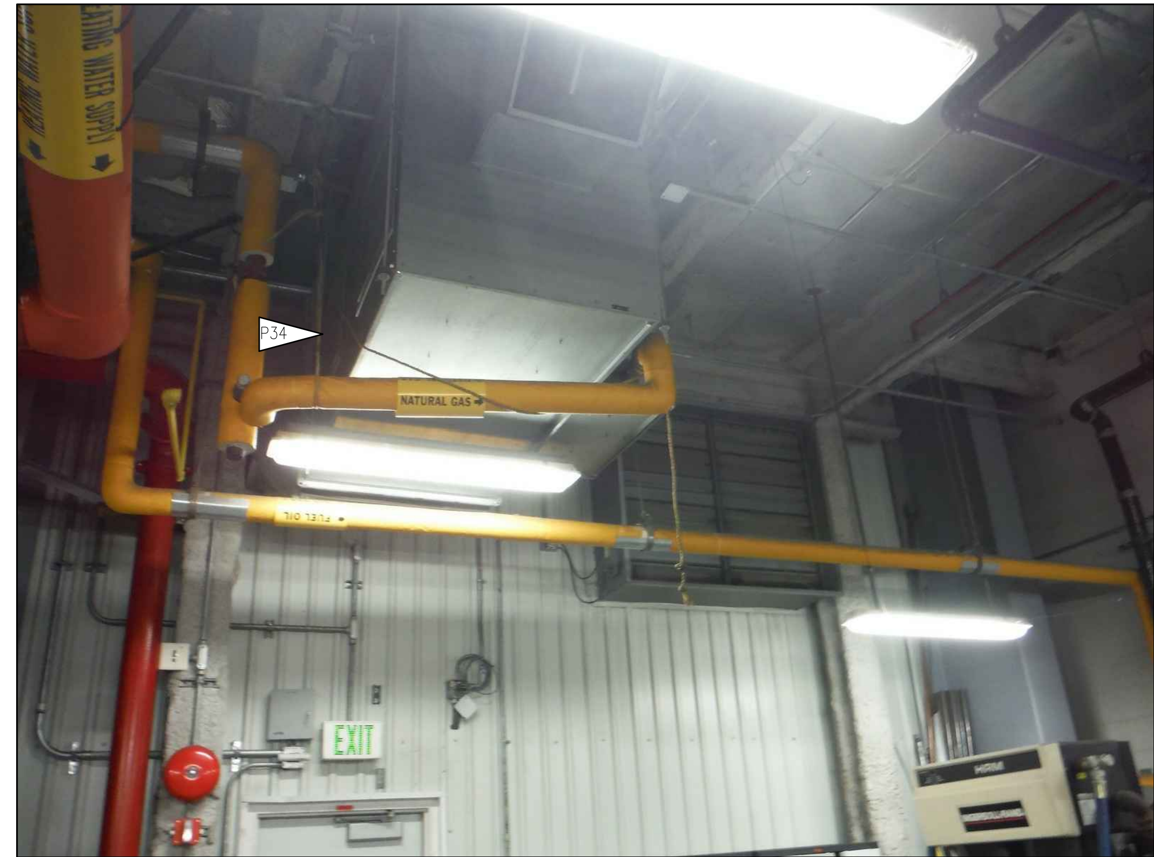
3 P34 - EXISTING MAKE-UP AIR UNIT AND DAMPER
