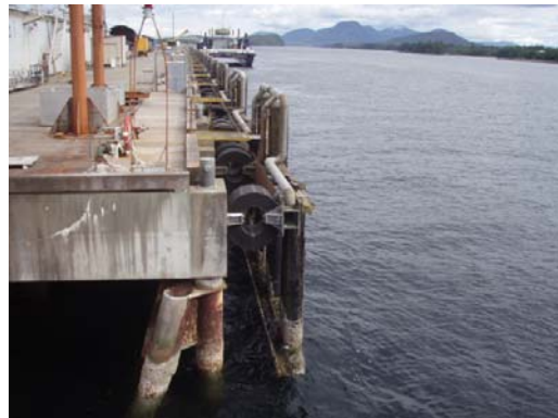
Fender on North end of North Pier
