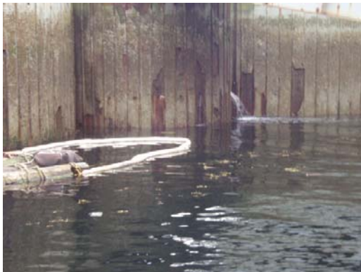
Interconnecting Arc Note drain hole
