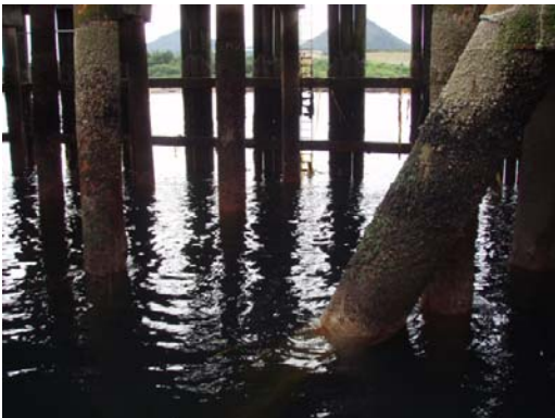
North Pier with fender in background
