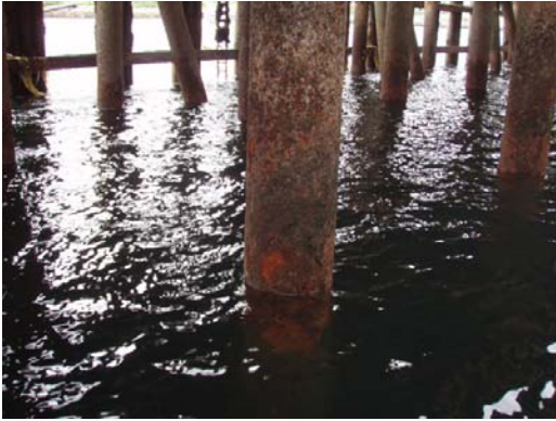
Typical North Pier Pile
