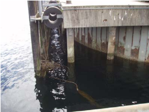
Fender on South end of South Berth
