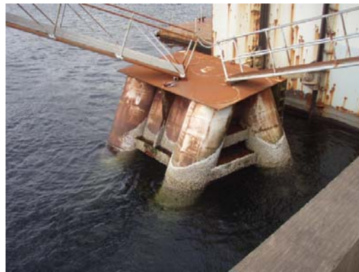
North Dry-dock Dolphin
