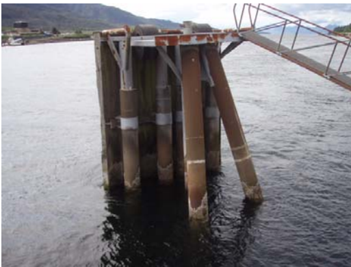
North Fender Dolphin
