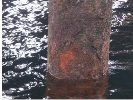
Typical North Pier Pile
