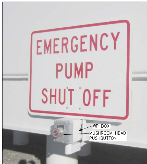
3 EMERGENCY STOP DISCONNECT (ESD) E6.01 SCALE: NTS
