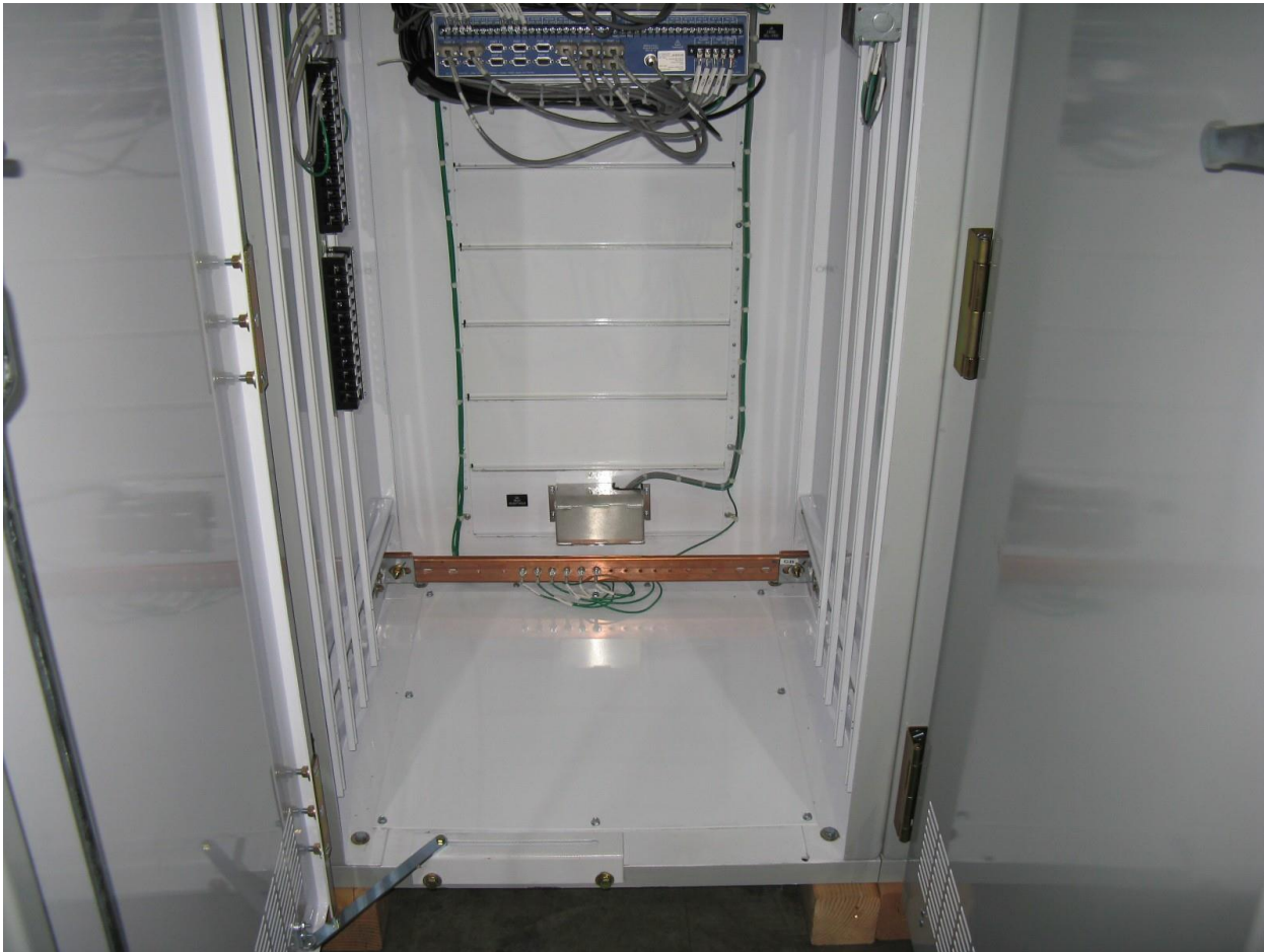
Figure 6: Typical Floor Mounting and Ground Bar
