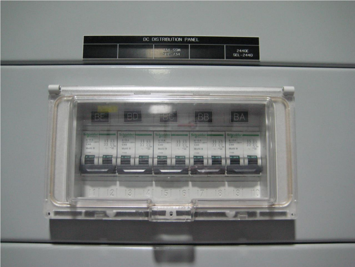
Figure 5: Typical Front View of a DC Mini-Breaker
