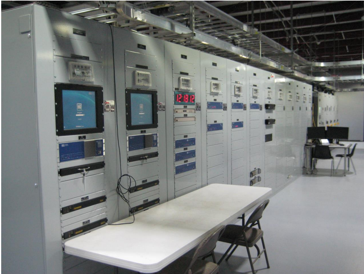
Figure 1: Typical Front View of a Relay Panel Line-up
