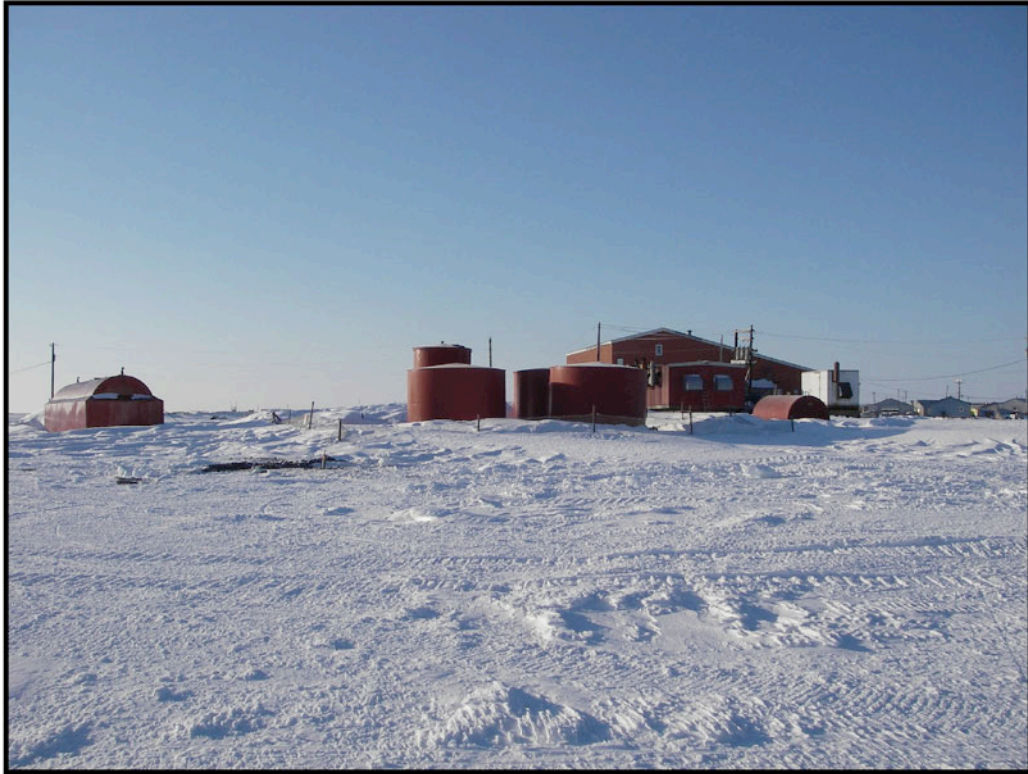
Existing Fuel Storage Facility and Corporation Offices, March 2007
