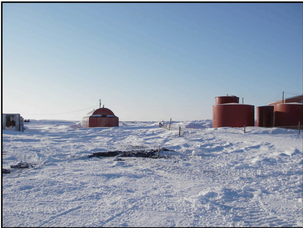
General Site Conditions, Kipnuk Fuel Tank Site, March 2007
