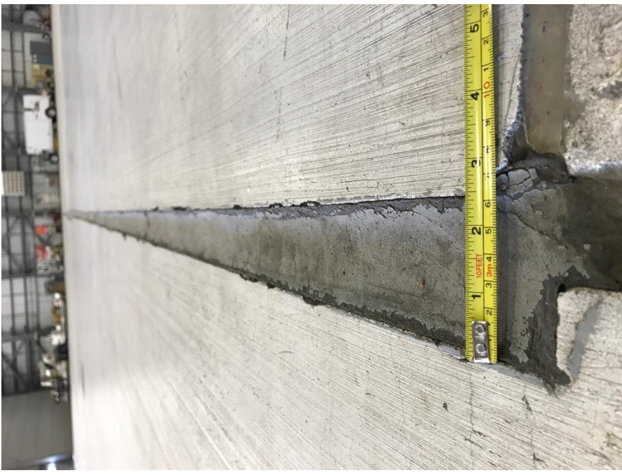
Photo 7 - Sealant deterioration and crack
