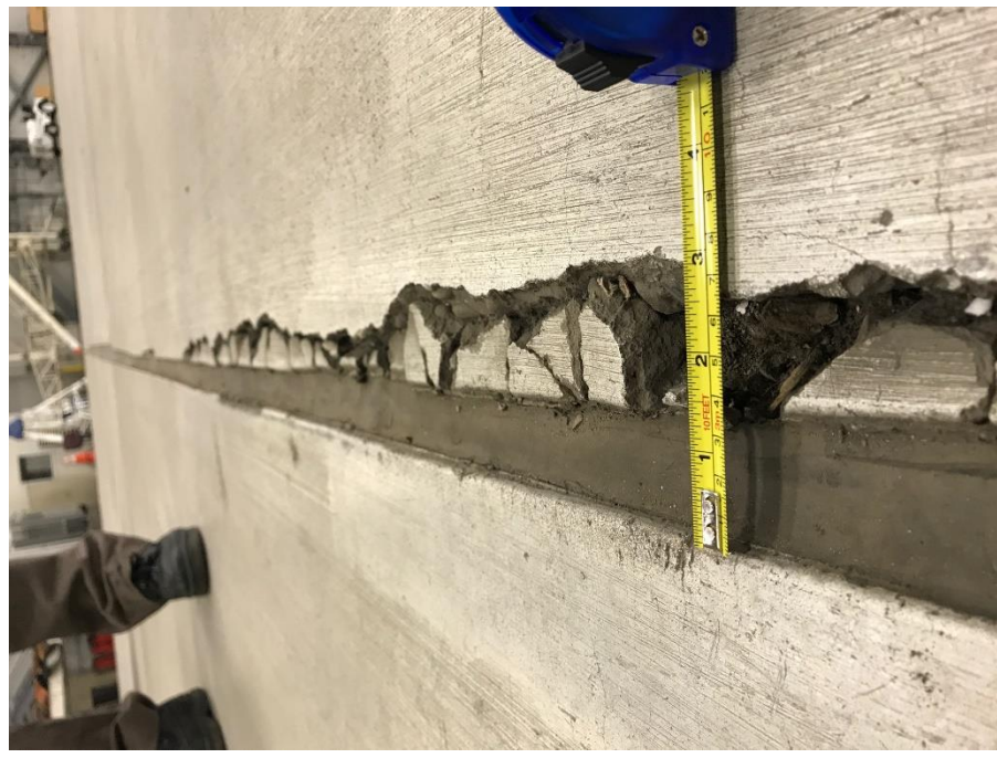
Photo 7 - Sealant deterioration and crack
