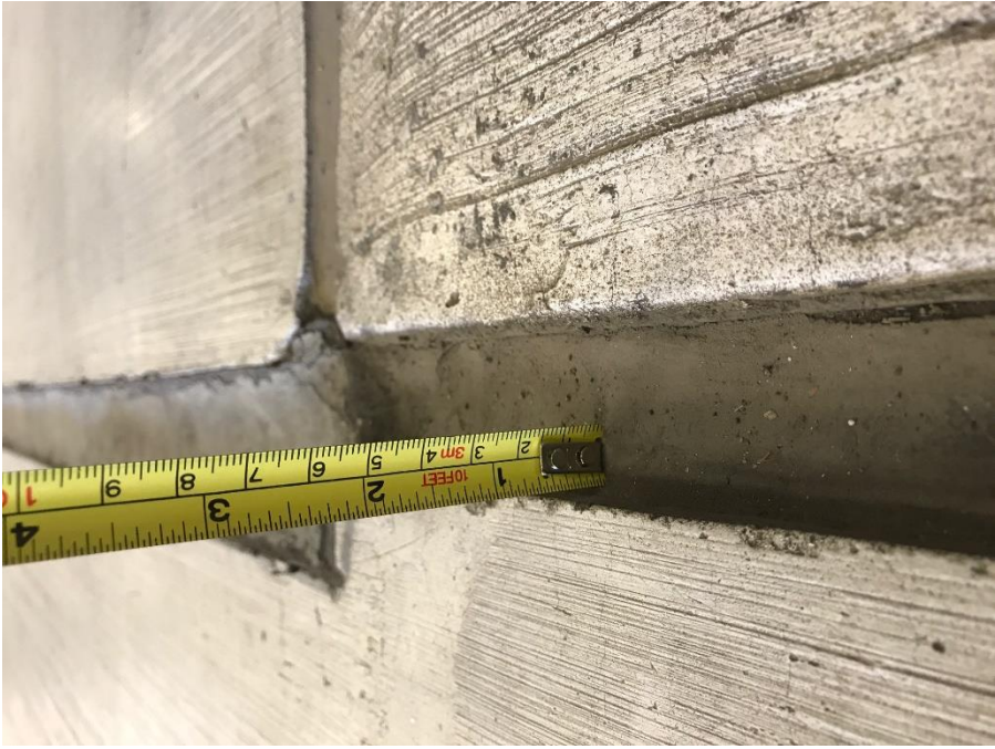
Photo 5 - Sealant shrinkage/settlement
