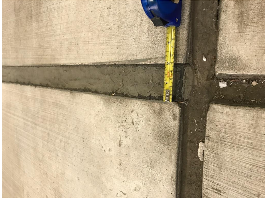
Photo 5 - Sealant shrinkage/settlement
