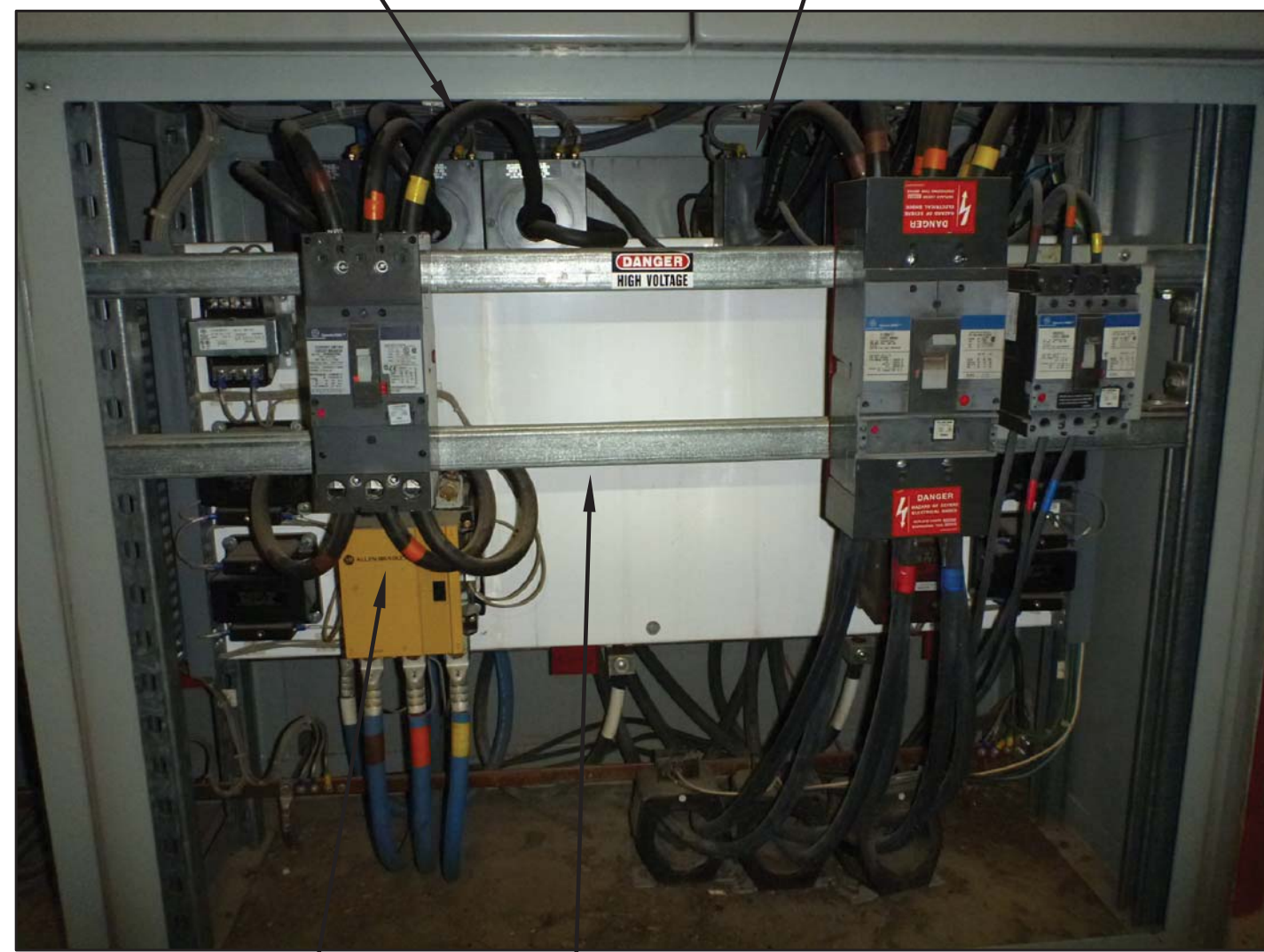
2 DIESEL PLANT SWITCHGEAR GEN #3 & FEEDER SECTION PHOTO E4 NO SCALE
