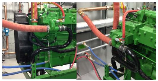
4. John Deere 6090AFM - Remove coolant expansion tank and other accessories that are not required. Manifold vent lines into a single connection near the front with a 3/8" NPT quarter turn gauge cock isolation valve. See photograph below for representative installation.
