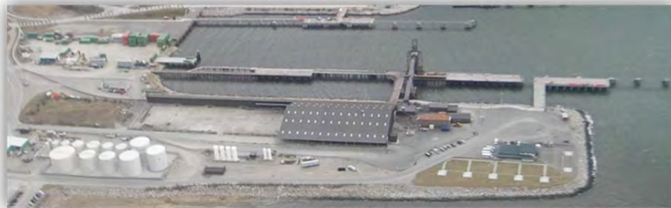
Aerial view of the Skagway Ore Terminal looking East
