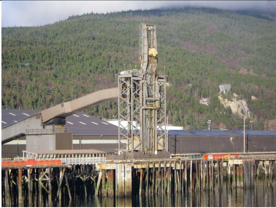
JM-111113-IMG0270 LOCATION: SKAGWAY ORE TERMINAL DESCRIPTION: VIEW OF SOT AND SHIP LOADER FROM THE WATER (STATE FERRY)
