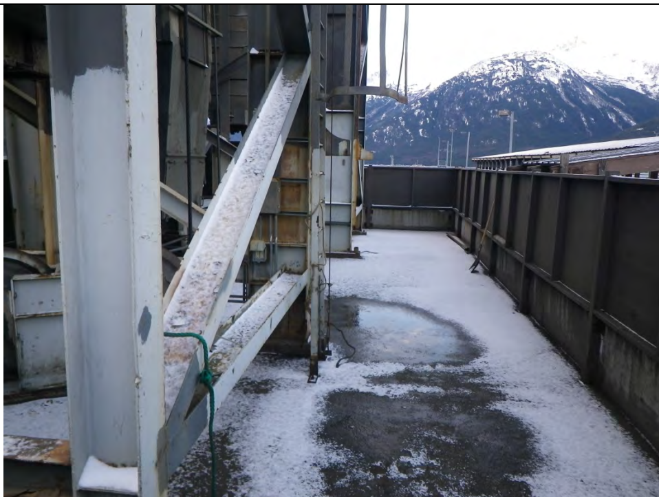
JKM-111313-IMGP0438 LOCATION: SKAGWAY ORE TERMINAL SHIP LOADER DESCRIPTION: FRESH SNOW AT BASE OF SHIP LOADER; VIEW FROM NORTH TOWER TO SOUTH TOWER ALONG WEST SIDE OF SHIPLOADER TOWERS
