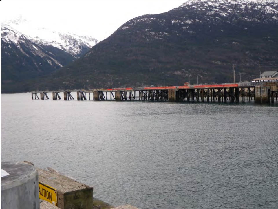
JKM-111213-IMG0429 LOCATION: SKAGWAY ORE TERMINAL ORE DOCK DESCRIPTION: ORE DOCK TO SOUTH OF SHIP LOADER AS VIEWED FROM ACROSS HARBOR
