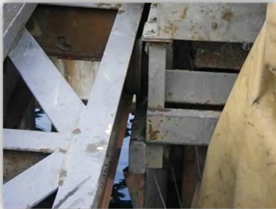
Right hand spout shuttle wheel, runway/track beam and failing lateral support.
