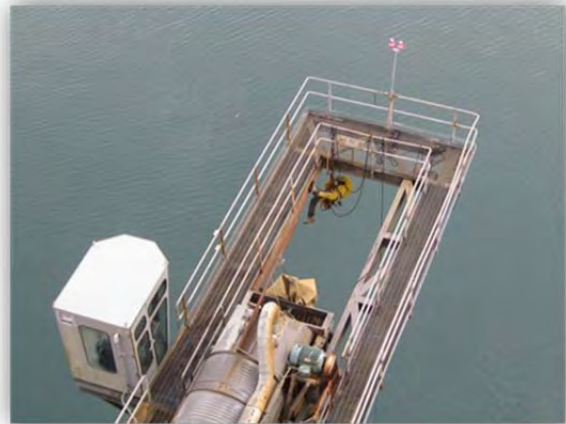
Right hand spout shuttle wheel, runway/track beam and failing lateral support.
