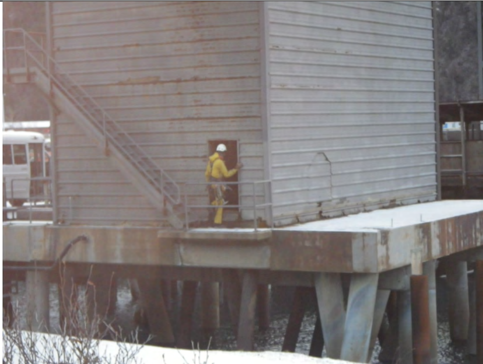
JKM-111313-IMGP0440 LOCATION: SKAGWAY ORE TERMINAL SHIP LOADER DESCRIPTION: INSPECTOR ENTERING DOOR AT BASE OF TRANSFER CONVEYOR MID-SPAN SUPPORT AND DRIVE TOWER
