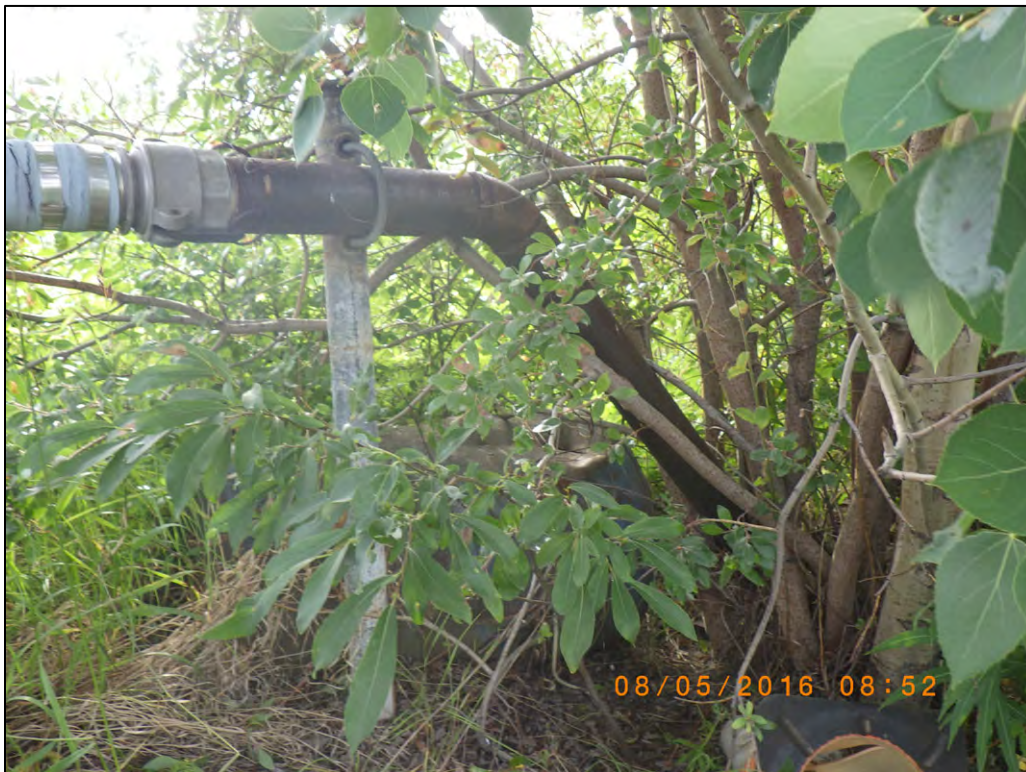
Photograph 2: Airstrip fill header
