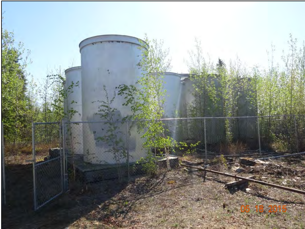
Photo 1 – School Tank Farm
