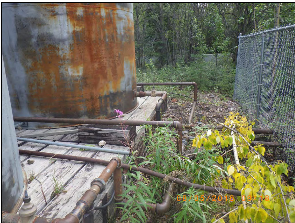
Photograph 8: Beaver Village tanks not-in-service at Tank Farm #1
