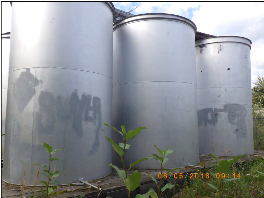
Photograph 3: Tank Farm #1; Cruikshank School and Village of Beaver tanks
