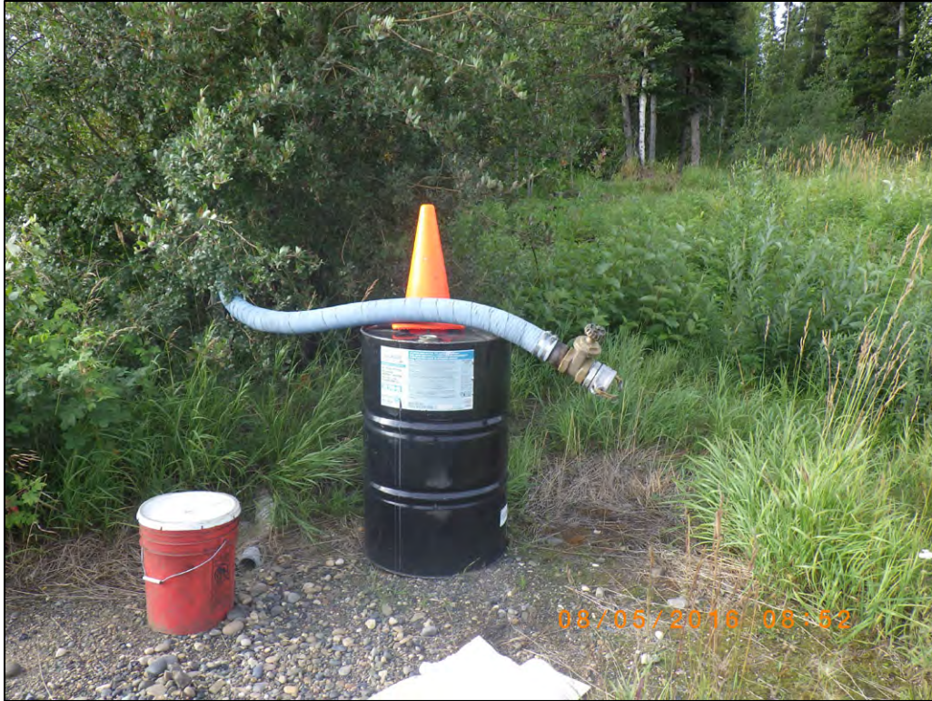
Photograph 1: Airstrip fill header
