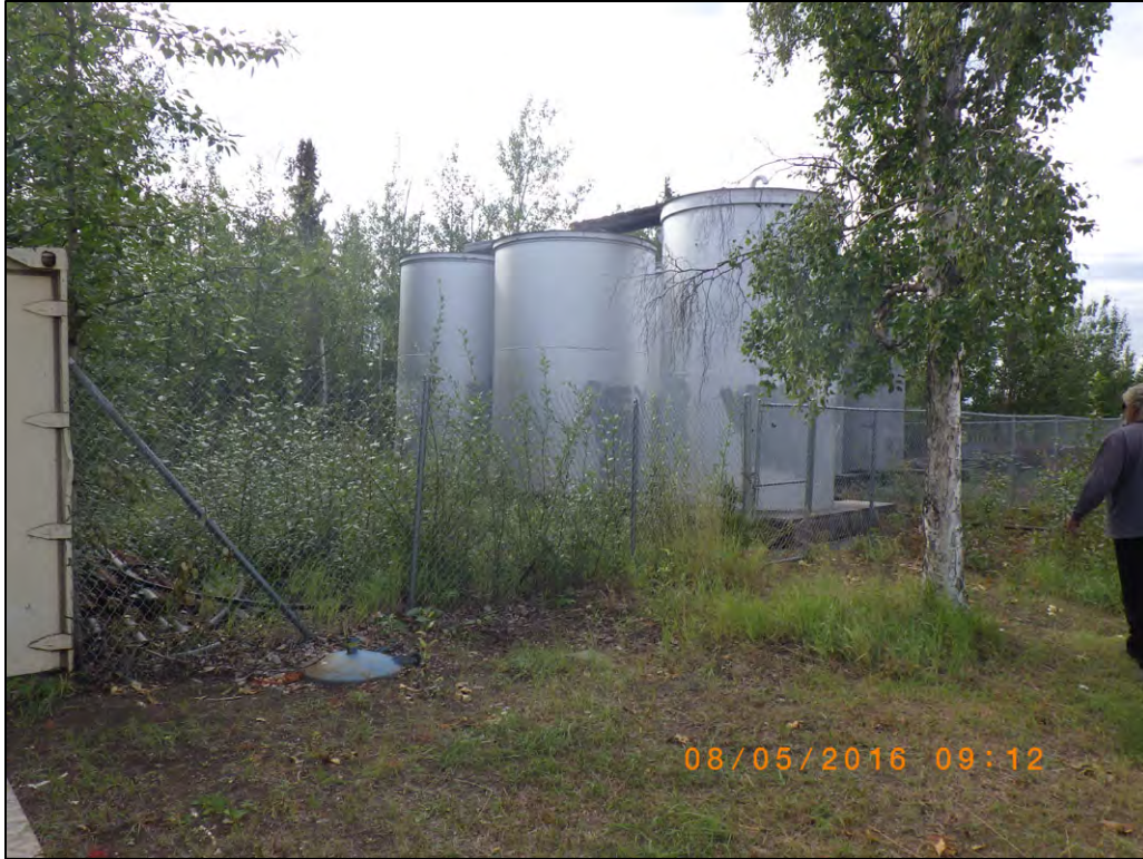
Photograph 2: Tank Farm #1; Cruikshank School and Village of Beaver tanks
