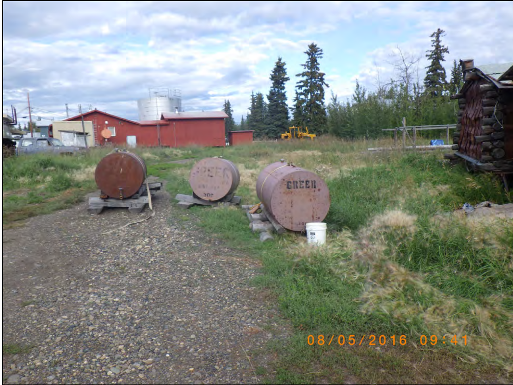
Photograph 15: 300 gal "Gasoline Shack" tanks on wooden skids
