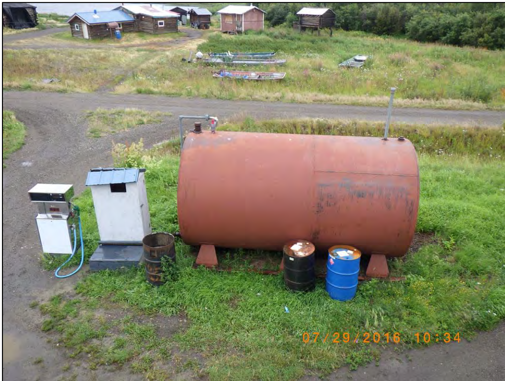
Photograph 10: Tank Farm #2 retail gasoline tank
