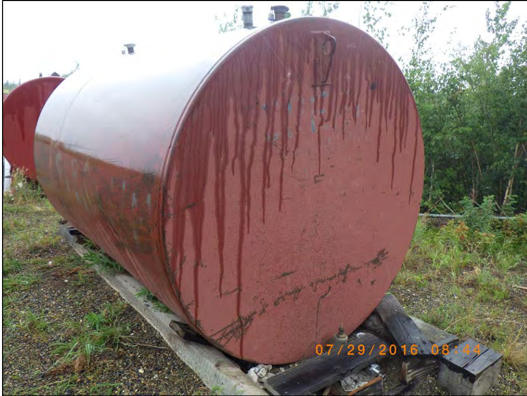
Photograph 15: Tank Farm #4 airstrip tanks
