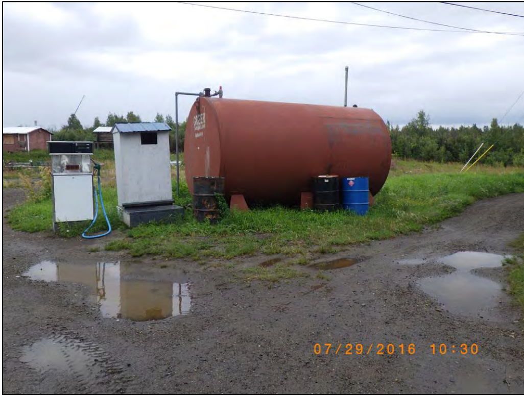
Photograph 9: Tank Farm #2 retail gasoline tank
