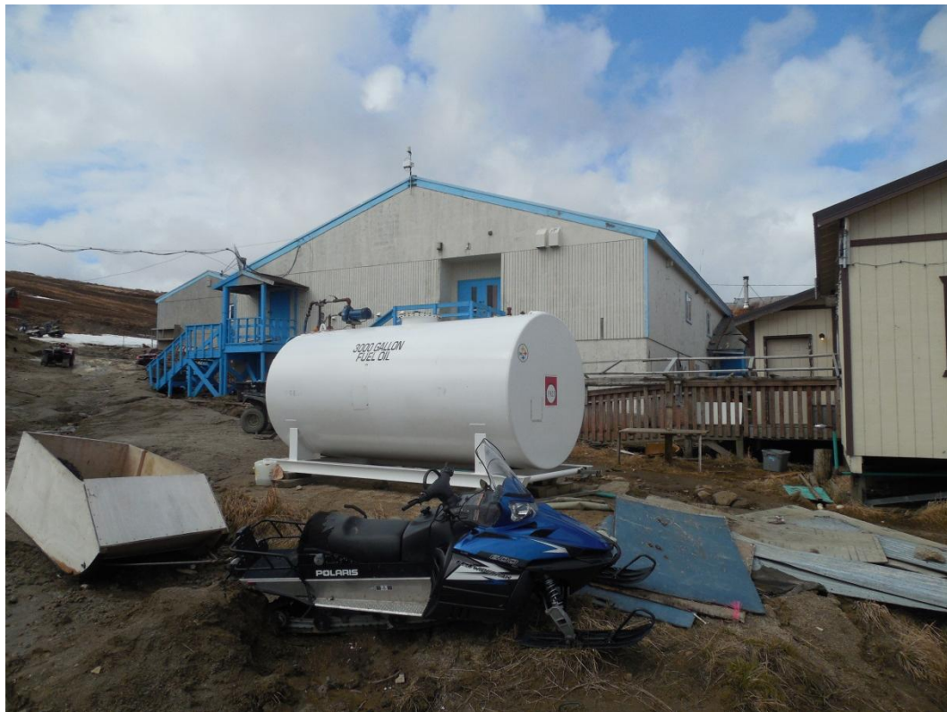
Photo 2 –City of Scammon Bay Office Tank Farm
