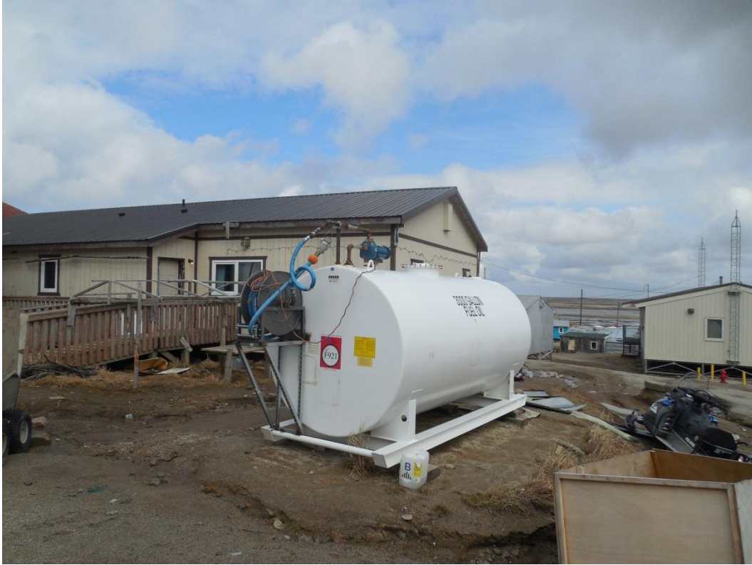
Photo 1 –City of Scammon Bay Office Tank Farm
