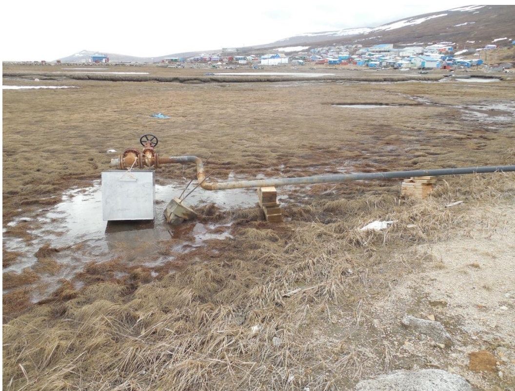
Photo 4 – Barge Header
