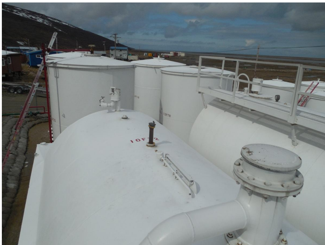
Photo 3 – Tops of Tanks
