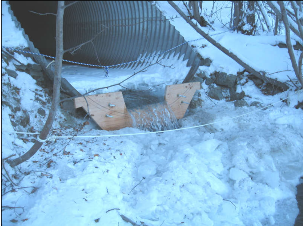
Photograph 1. Lower weir installed at culvert outlet. CEI, January 7, 2008.
