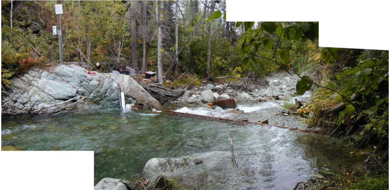
Photograph 5. Newly completed upper weir gauging station. Polarconsult. August 28, 2009.
