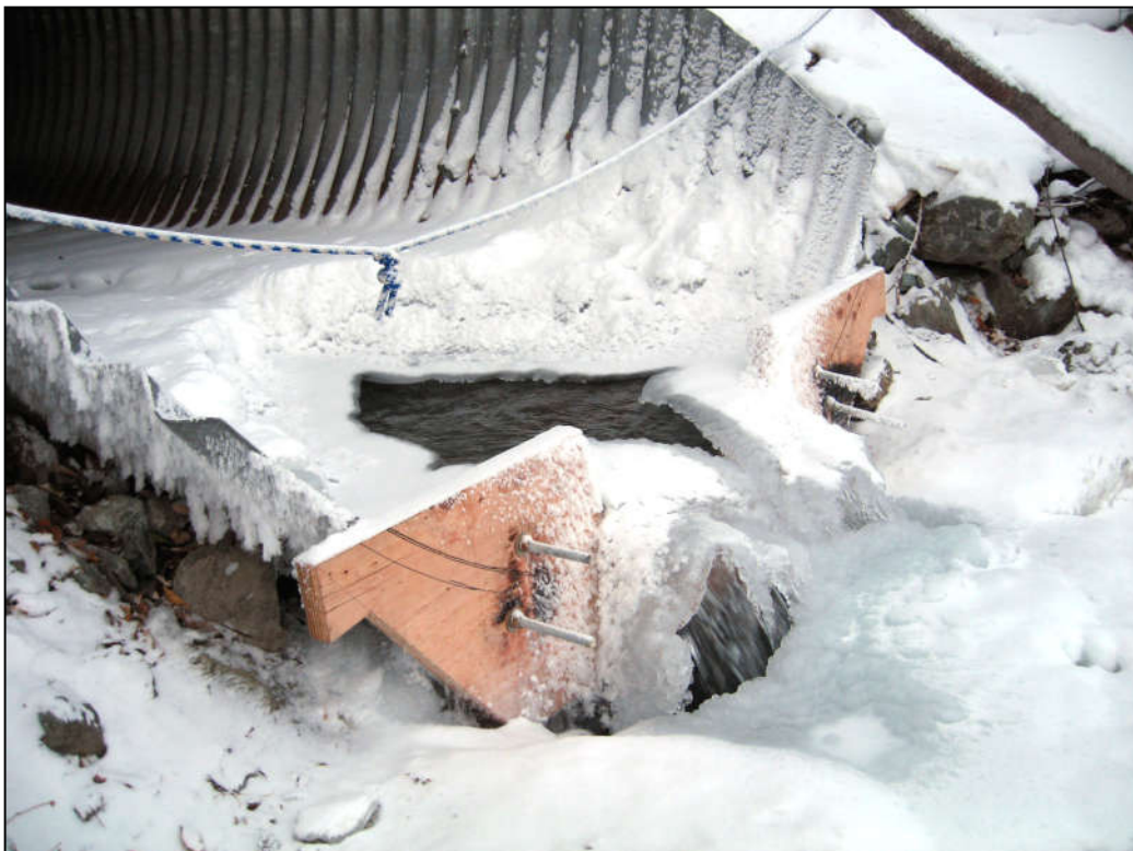
Photograph 2. Lower weir installed at culvert outlet. CEI, January 9, 2008.
