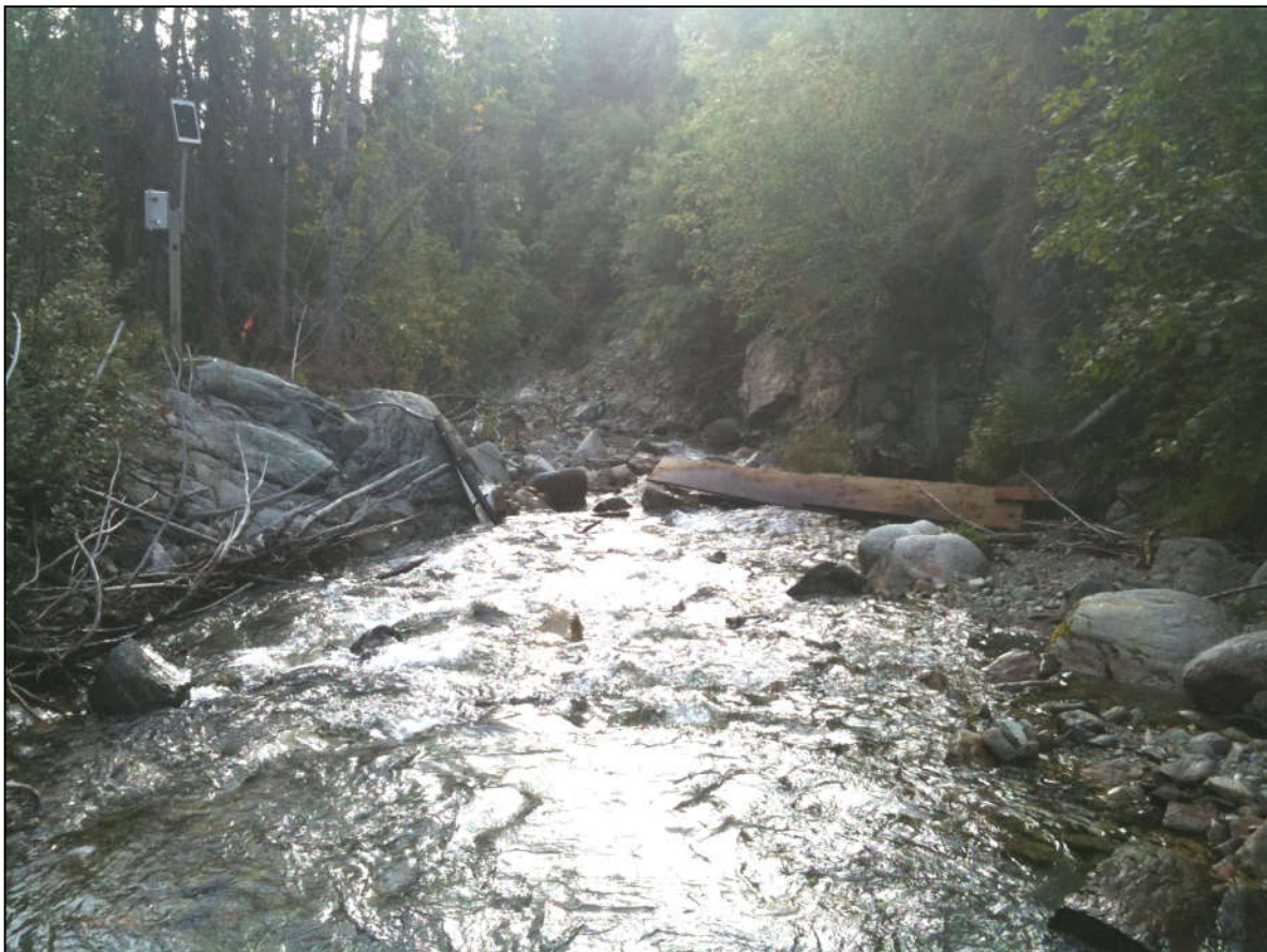
Photograph 6. Upper weir gauging station after weir failure (downstream view). Polarconsult. August 20, 2010.
