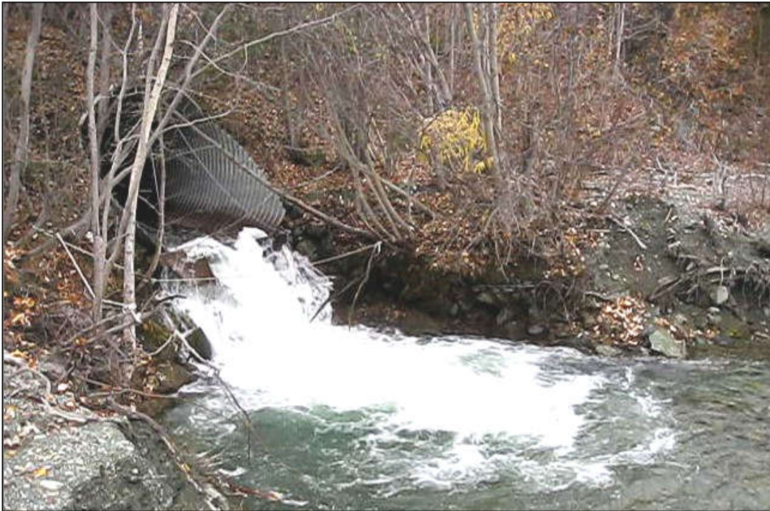
Photograph 3. Lower weir installed at culvert outlet. CEI, October 13, 2009.
