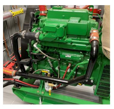
2. 6068AFM - Remove coolant tank and other accessories that are not required. Modify coolant discharge connection to face vertically at the front of the engine. Modify coolant suction connection to face horizontally at the front of the engine. See photograph below for representative installation.
