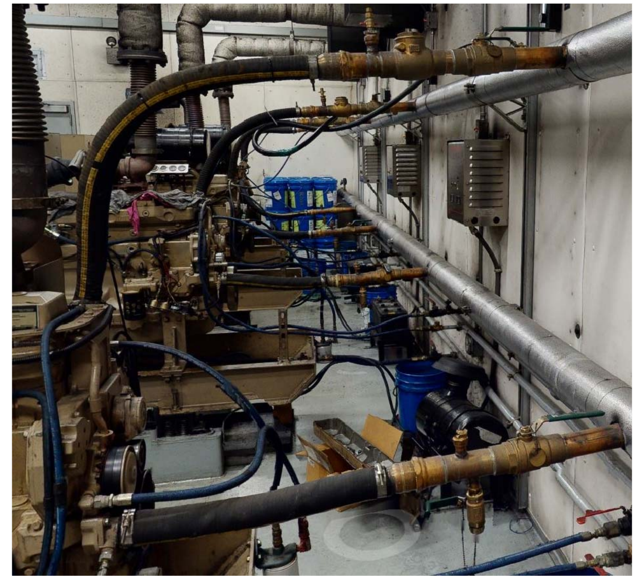
2 TYPICAL EXISTING ENGINE COOLANT HOSES M4 NO SCALE
