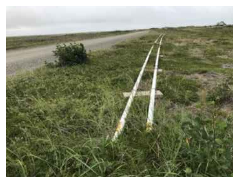
PIPE FLANGE CONNECTION APPROXIMATELY 150-FEET FROM BARGE HEADER
