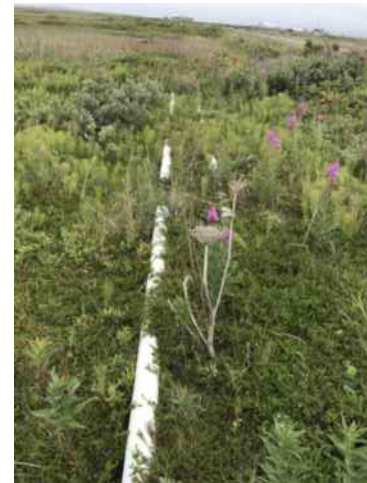
ABOVE GROUND PIPE
