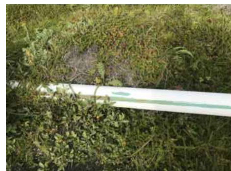
ABOVE GROUND PIPE COATING DAMAGE
