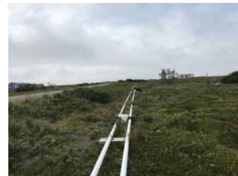
PIPE FLANGE CONNECTION APPROXIMATELY 300-FEET FROM BARGE HEADER
