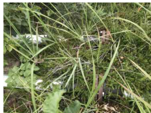
PIPE FLANGE CONNECTION APPROXIMATELY 150-FEET FROM BARGE HEADER
