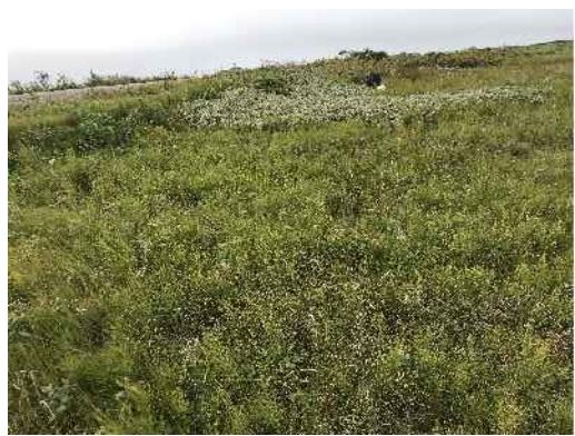
ABOVE GROUND PIPING - SUNKEN INTO TUNDRA
