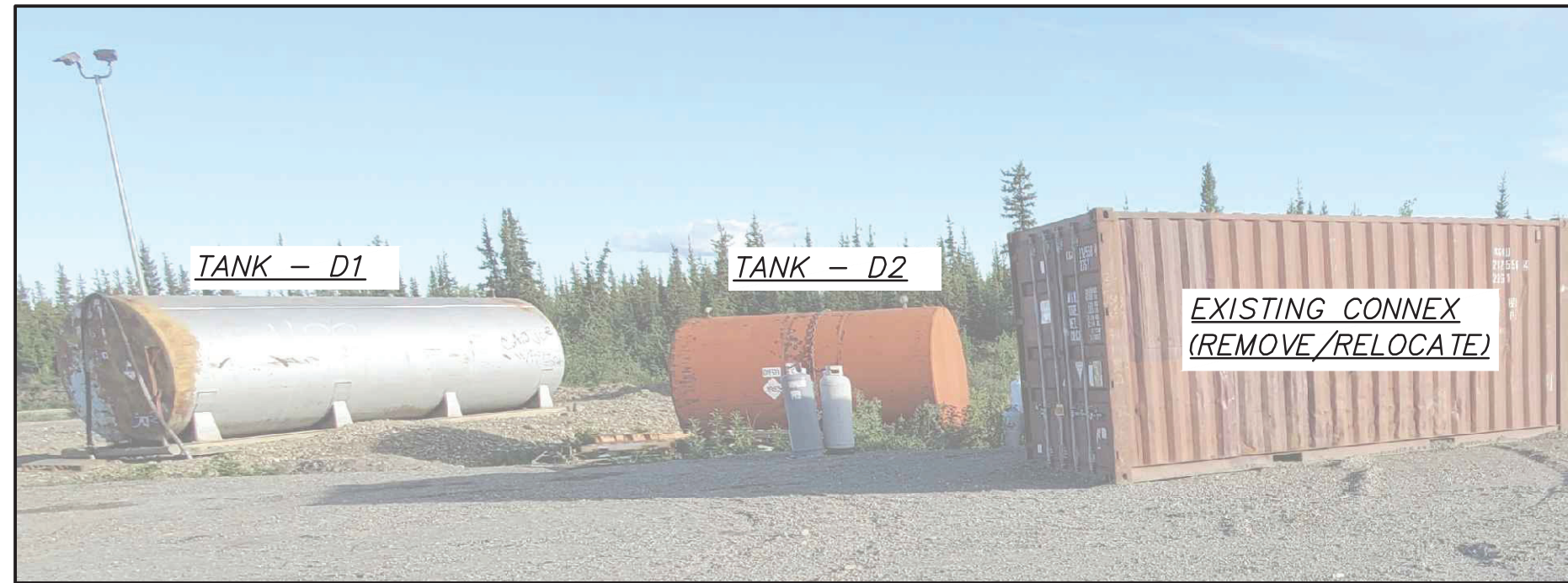
PHOTO # 1 : TANK FARM SITE AT VENETIE AIRPORT, SUMMER 2021
