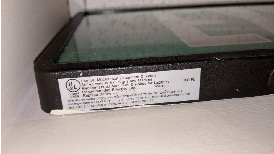
Self-luminous exit sign
