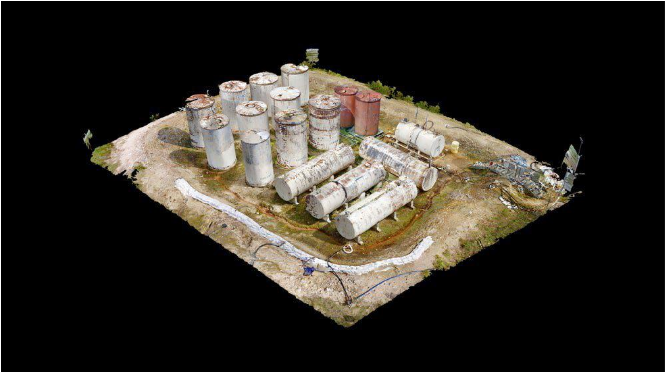
Example Remote Bulk Fuel Tank Farm (Use outdoor camera)
